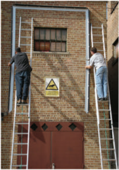
Mounting frame sides to our building.
