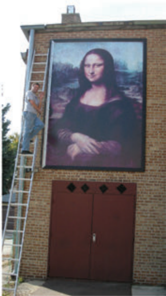
Clamp tightening finished, frame sides closed, 90 minutes total installation time.
