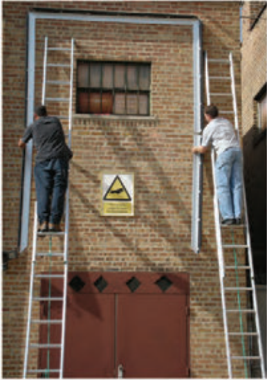
Mounting frame sides to our building.
