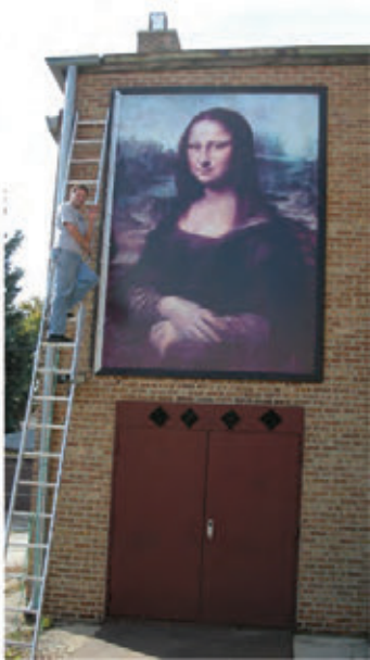
Clamp tightening finished, frame sides closed, 90 minutes total installation time.
