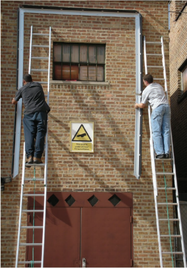
Mounting frame sides to our building.
