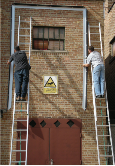
Mounting frame sides to our building.
